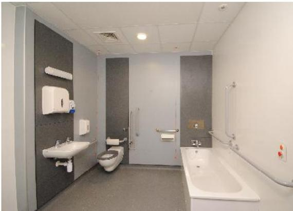
Further to value engineering, the system provided consisted of a mixture of timber and metal framing, faced with solid grade laminate panels. The system was delivered to site as a two-part process, allowing the ceilings, whiterock and flooring to progress while leaving the pre-plumbed panels off-site for a final fix operation.
